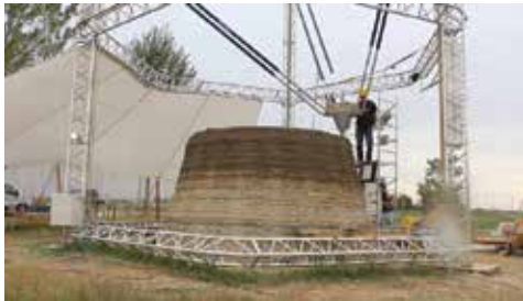
Exposed (unregulated) curing environment *4
