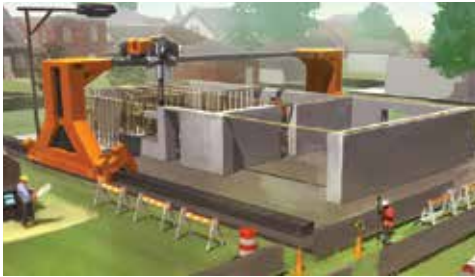
Large heavy 3D Construction systems with complex setup (requires a crane) *1
