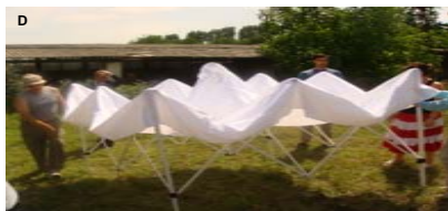
D. It takes at least two people to set up the Pop up tents: gently pulling at the corners to extend the supports.
