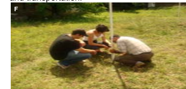
F. Stakes are driven into the ground at each leg to secure the structure against winds. The tents prepared in this way can withstand many weather conditions.
